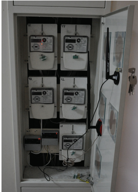
Fig. 12. Energy meter case with installed ZigBee adapters
