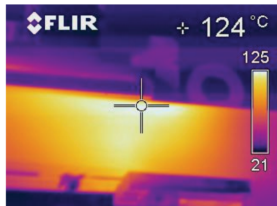
Fig. 8. Electromagnetic interaction of a planar busduct: a) steel structure of the electrochemical equipment housing provided with planar busducts; b) thermovision picture of the (a) system
