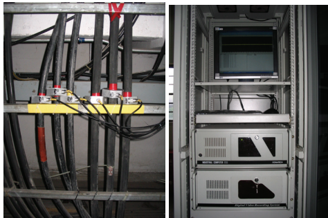
Fig.3. Online PD monitoring system for subway cable.
