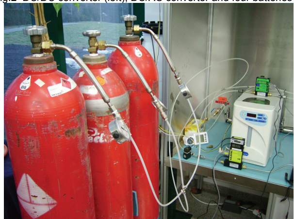
Fig.3 Pressure vessels to store hydrogen produced by the electrolyzer (right)
