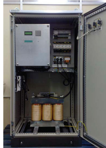
Fig.9. Equipment for inductor tests
