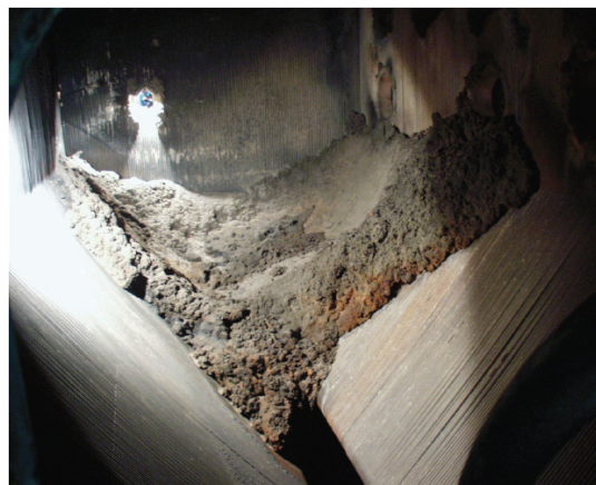
Fig. 6. Clogged slug removal funnel [10]
