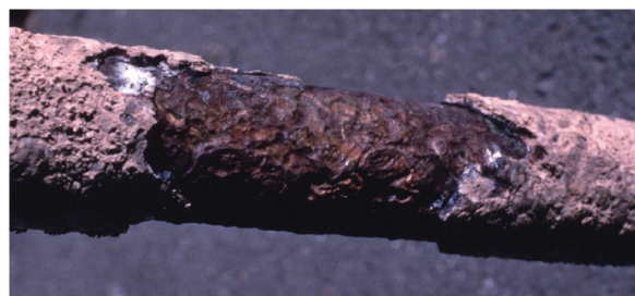
Fig. 7. Corrosion of a biomass boiler superheater tube after two years of service firing high chlorine fuels [11]
