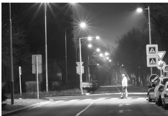
Fig.1. Photography of pedestrian crossing – luminaire MACH1
