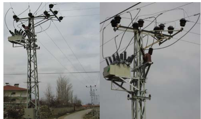
Fig. 4. The installed figure of the NGR on line at Gölbaşı district of Ankara, Tuluntaş/Oğulbey neighbourhood.
