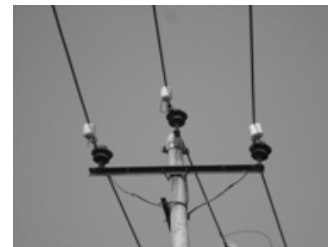
Fig. 4. Detection device installing picture
