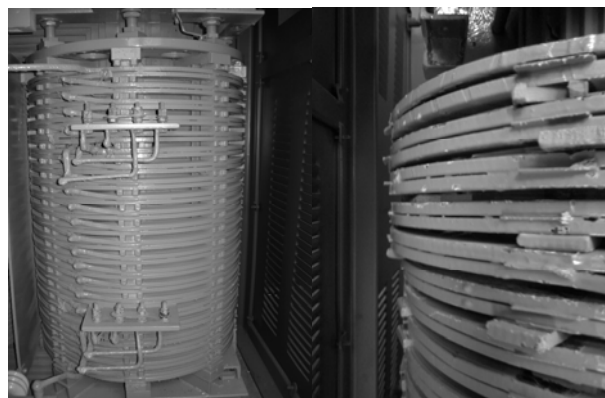
Fig. 1. The view of test winding (left) and an example of a radial deformation (right)
