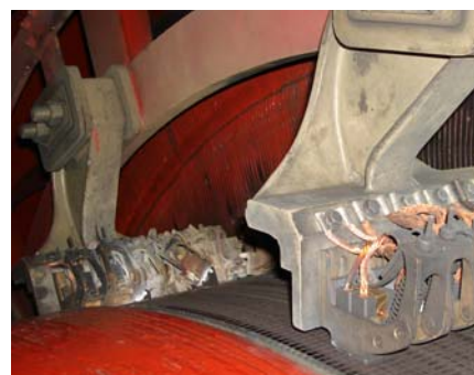
Fig.2. Damaged brushes of one of the polarities in a roller machine
