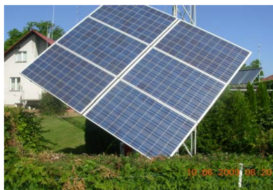
Fig. 2. Example of photovoltaic installation provided with Sun follow-up; the tracker with PV modules without the concentration system 2-axis, the Communication Plant of Alarm System PHU, Leżajsk (Poland), with approval of Mr. Stanisław Krupa
