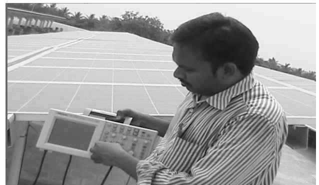
Fig.13 Leakage current measurement in the field
