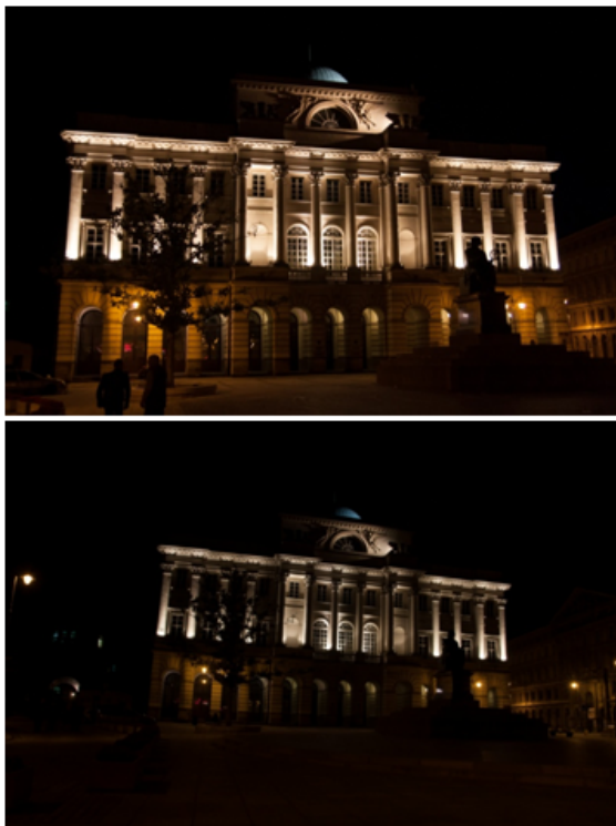
Fig.1. Staszic Palace in Warsaw floodlighting (without cropping and post processing)
