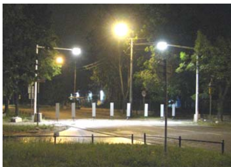
Fig. 12. Light frames type 2 permanently installed on pedestrian crossing
