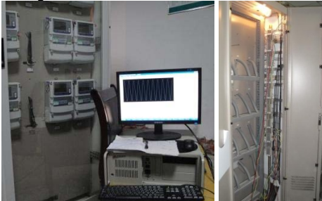
(b) On-line monitoring system operating in field
