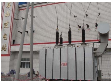
(a) Testing transformer in Shishan transformer substation
