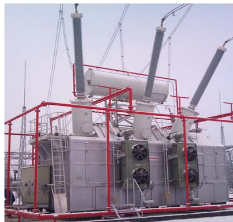
Rys.1 Autotransformator ANSR3L 250000/400PN
