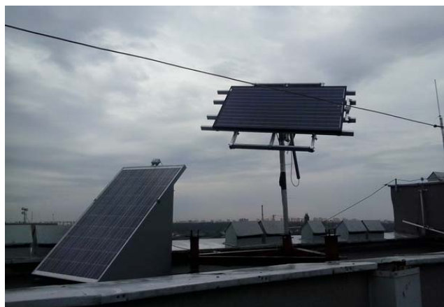
Fig.2. A view of the measurement stand consisting of a 2-axis tracking system and a fixed system located on the roof of the Institute of Electrical Engineering of Poznan University of Technology
