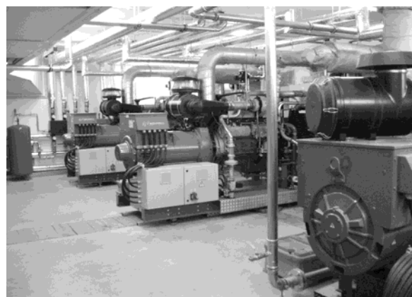
Fig.1. Co-generation units: 2 x 250 kWe and 1 x 340 kWe
