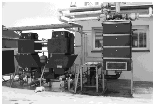
Fig.2. Biogas quality alteration device (dehumidification and desulphurizing)
