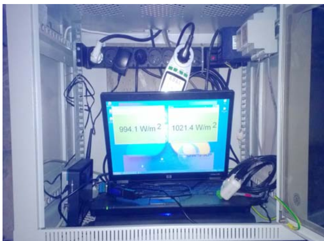
Fig.5. Equipment of photovoltaic system consisting of overvoltage reduction unit, computer, gateway modem and supply
