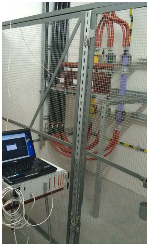
Fig.2. Test stand for measurement of current decay in the generator armature winding located in the excitation room of Mikołaj Power Plant
