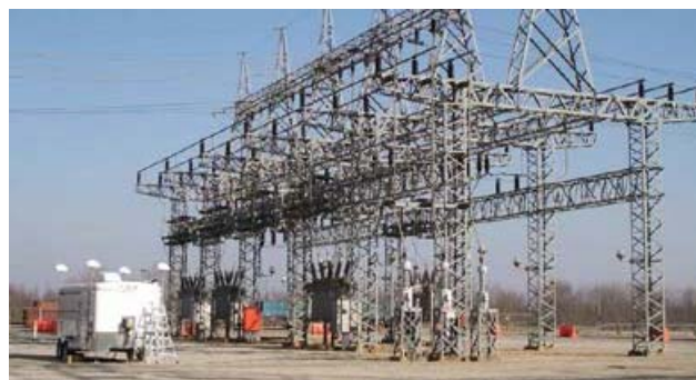
Fig.2. TVA early warning system installation
