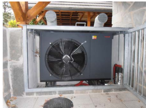
Fig.1. Installed heat pump (Šrámek, 2012)
