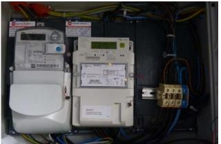
Fig.6. Pilot site – electric energy meter for electricity production and consumption
