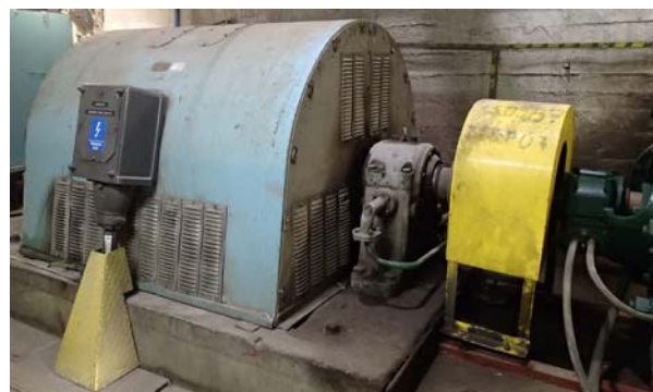
Fig. 9. The existing drive of the main mine drainage using the asynchronous motor type SBud 154d
