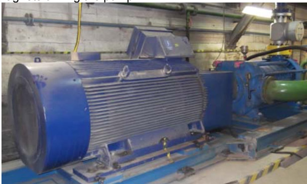
Fig. 10. The prototype synchronous motor with permanent magnets mounted on the workstation driving the main mine drainage pump
