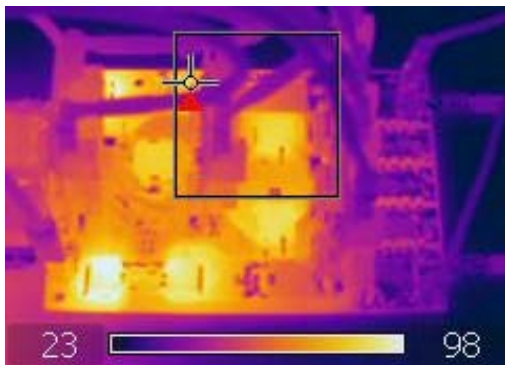
Fig.12 IR Thermograph of the converter operating with maximum power. The hottest points are the diodes. Steady state at 300W operation.
