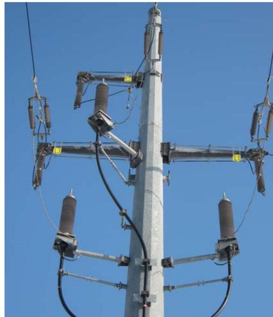
Fig. 1. High voltage 110 kV transmission tower covered by the installation of UHF sensors
