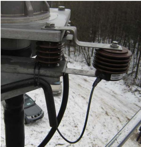
Fig. 3. The method of assembly the UHF sensor to the cable termination
