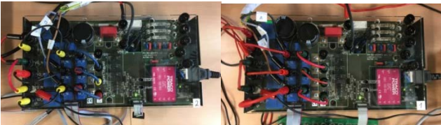
Fig.13. Applied P4-50-600 MFE frequency converters
