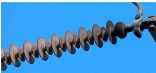
Fig.13. Pollution accumulation near the high voltage flange of the composite insulator [32]
