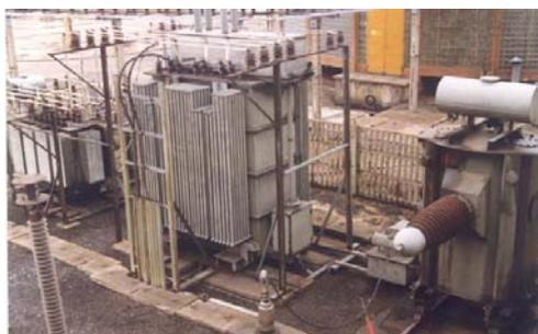
Fig. 3. Supply transformers. From left to right: the symmetry transformer (supplied by three 6 kV phases), regulation transformer and high voltage transformer 6/200 kV.
