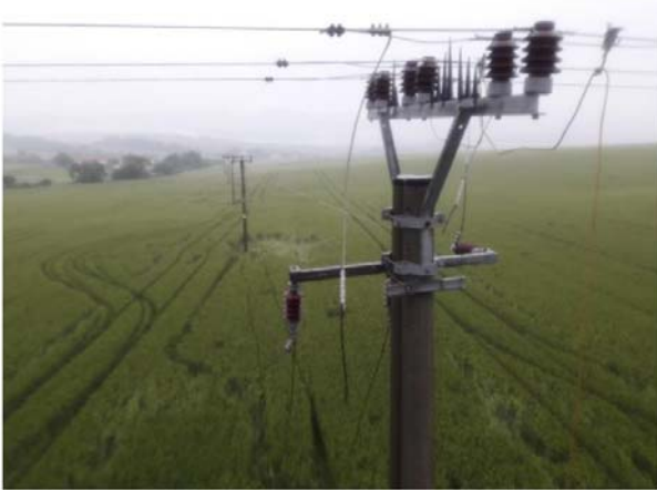
Fig. 20. Damage caused to the overhead line after a breaker failure – 2 downed conductors
