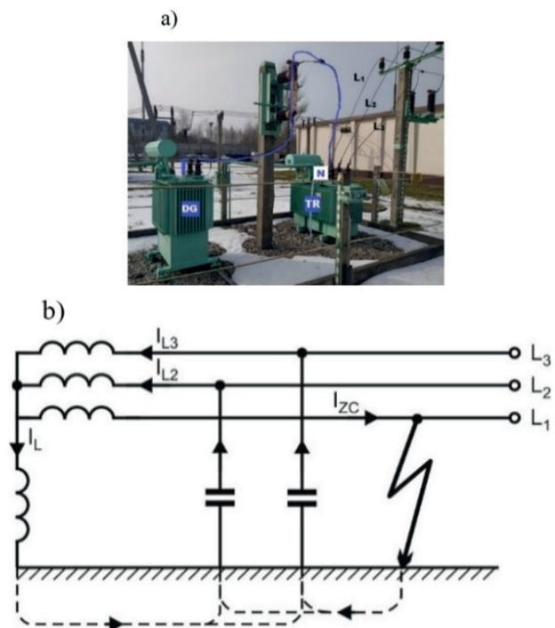
Fig. 5. Ground fault current compensation: a) a view of DG arc-suppression coil connected to N point of transformer TR, b) current distribution during ground fault with compensation
