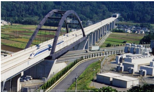
Fig. 19. Yamanashi Maglev Test Line: Ogotayama Bridge over the Chuo Expressway. Public domain photo.
