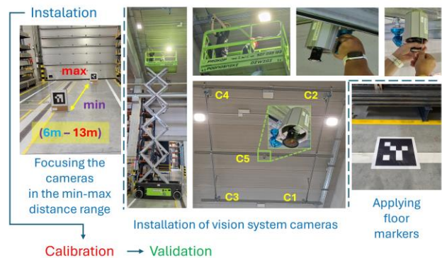
Fig. 7. Commissioning of the vision system on the target measurement stand – installation
